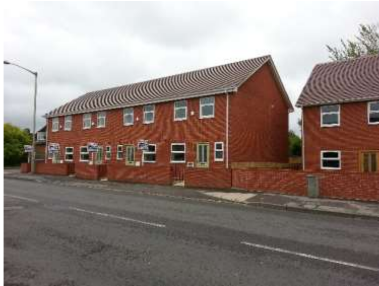
New build flat façade, gives dull appearance, Cheltenham Road Estate
