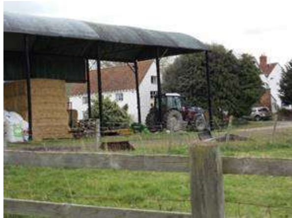
Pirton Court – old farm buildings with steeply pitched roofs, small windows
