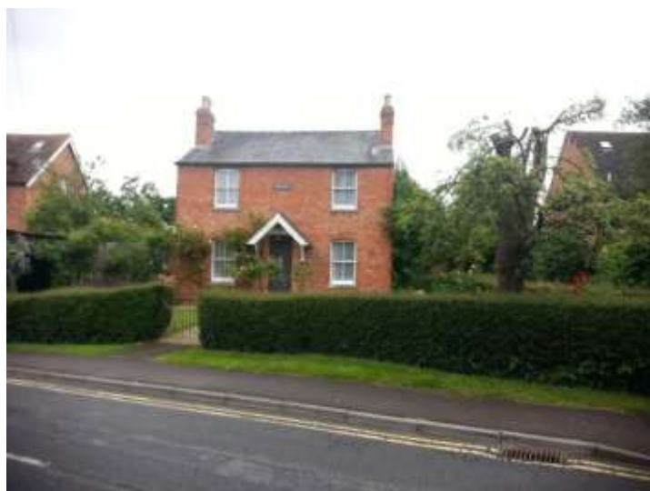
Old Farm House, Brookfield Road
