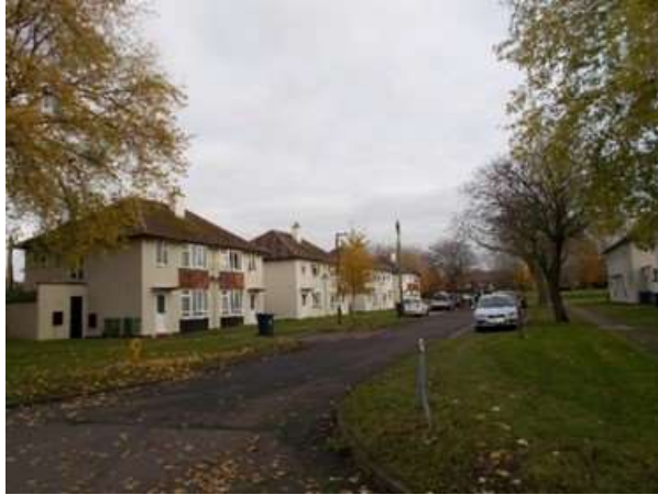
Characteristic red and white/off white, use of red tiles lifts the appearance, Mottershead Drive, Innsworth (housing for military families)
