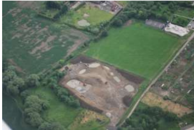
Overview of Churchdown Park during ponds construction, showing field, MUGA, skatepark
