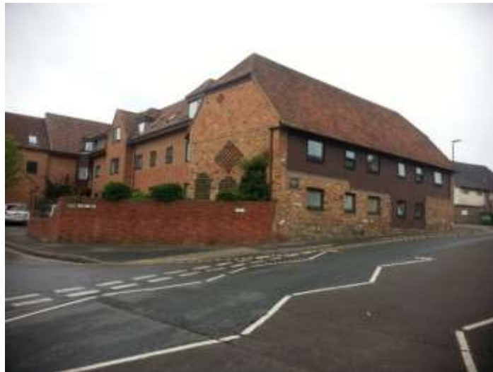
Sweetbriar House, Chapel Hay Lane, built in style of old farm buildings as shown below – use of variegated brick and replica elm boards in style of old farm building
