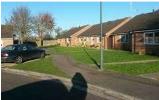
Open front boundaries are low maintenance, and present open, uncluttered appearance, Chaffinch Close, Innsworth
