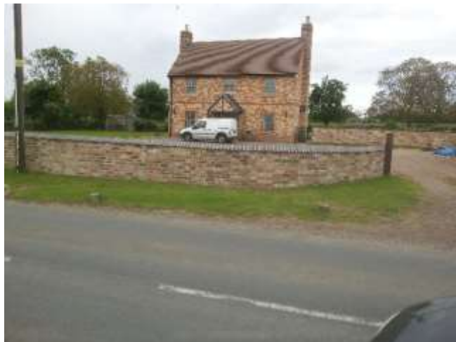
Woodlands Farm - old farmhouse rebuilt using old variegated brick and new. Very characteristic of the local brick made from clay dug out in field nearby (Brockworth Road, Churchdown)
