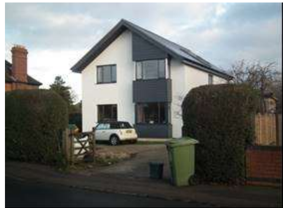
Modelled façade on modern house, Parton Road, Churchdown
