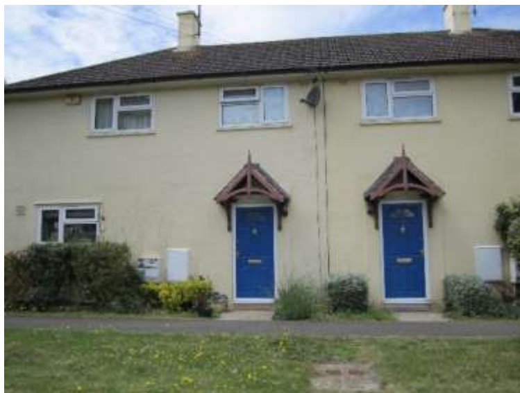
Later addition of porches to relieve flat façade, Innsworth Lane, Innsworth
