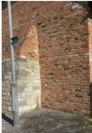
Variegated brick at Sweetbriar House, Chapel Hay Lane
