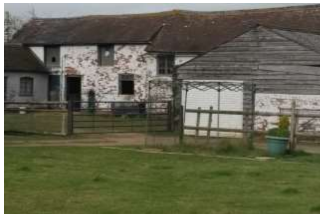
Innsworth House Farm – traditional farm building with steeply pitched roofs, small windows and elm boarding
