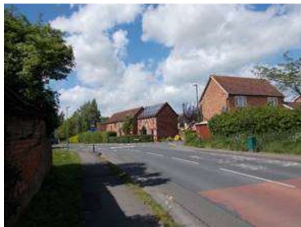
New Build, Pirton Meadow, opposite old buildings of Pirton Court, the new design reflects the older farm buildings and is pleasing
