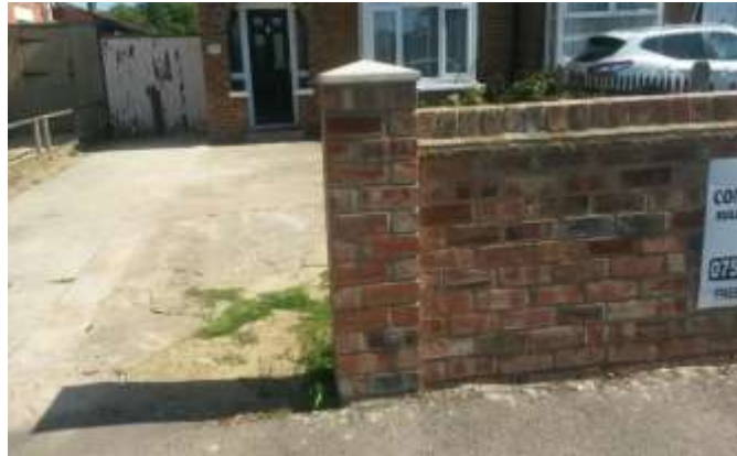
Variegated brick used in new wall, Pirton Lane
