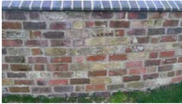
Close up of variegated brick at Woodlands Farm
