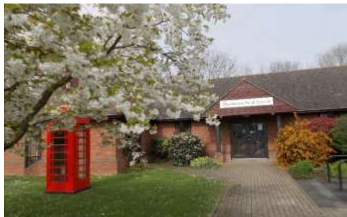
Churchdown Parish Council Offices
